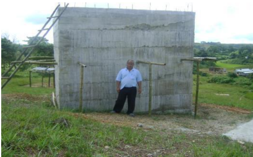
Photo 7.5 Construction of community tank in progress in JaintiaHills
