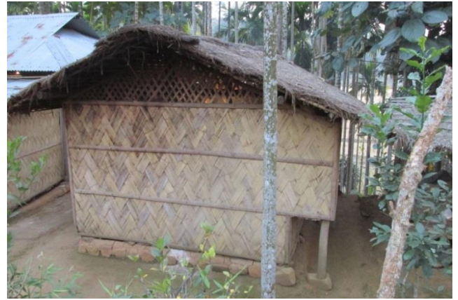
An old Hut of the beneficiary
